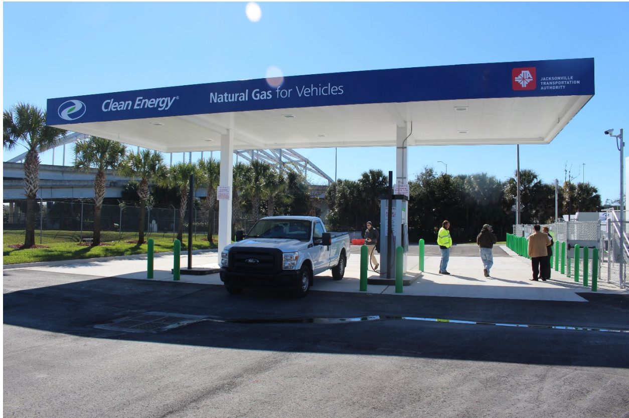
FIGURE 2: JACKSONVILLE TRANSPORTATION AUTHORITY'S PUBLIC CNG STATION
