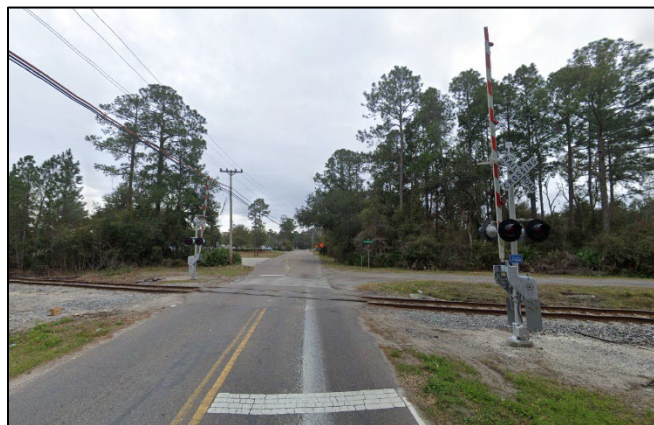
Existing railroad crossing. Photo Source: Project Team.
