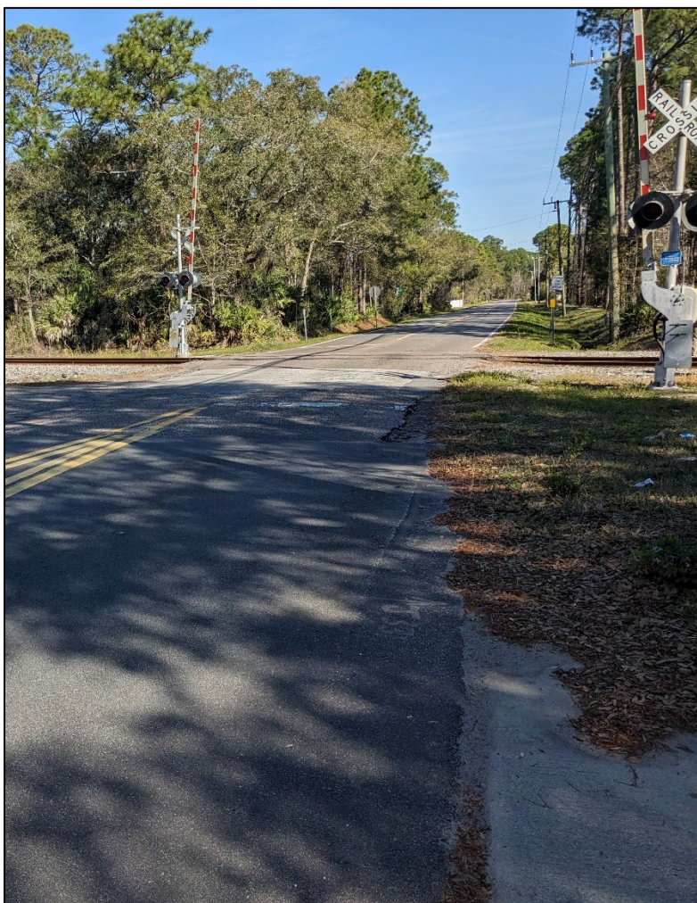
Railroad crossing. Photo Source: Project Team.
