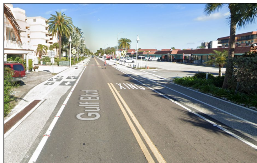
Example of a Pedestrian Bicycle Lane (SR 699, Indian Shores). Photo Source: Project Team.
