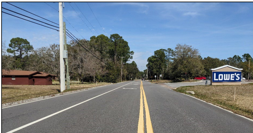
Commercial development (Lowe’s) on southern end of the corridor. Photo Source: Project Team.
