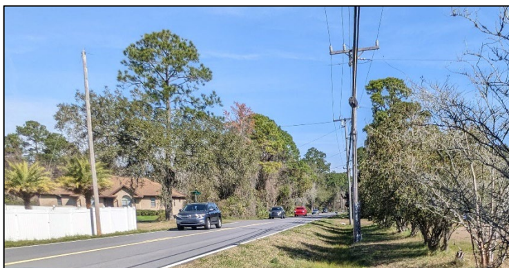
Utility poles near ROW. Photo source: Project Team.
