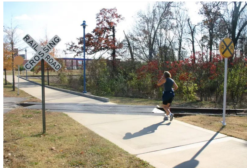
Example Shared Used Path Crossing without Gates. Photo Source: American Trails.
