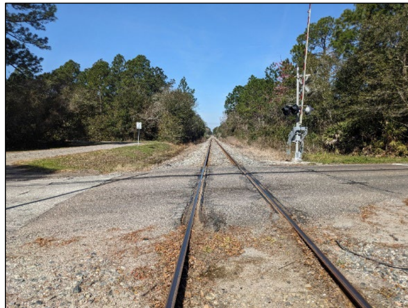
Existing railroad crossing. Photo source: Project Team.
