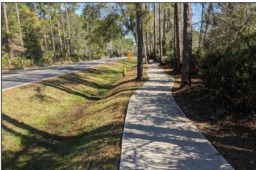
Existing sidewalk segment. Source: Project Team.
