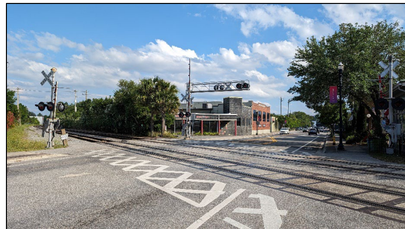
Example RR Crossing with Pedestrian Gates. Photo Source: Project Team.
